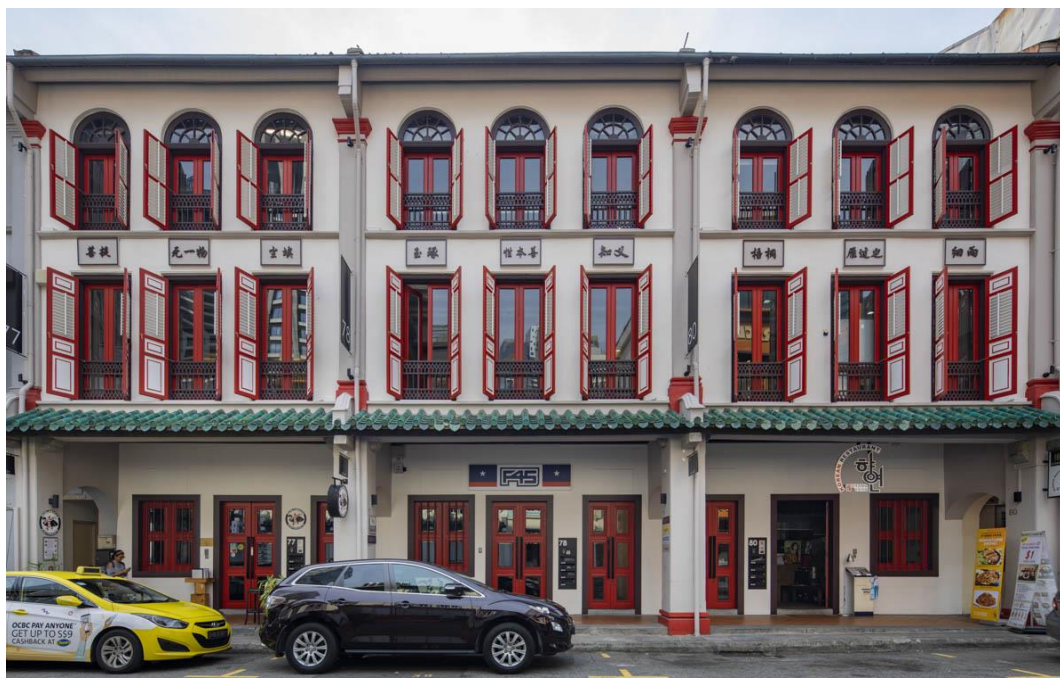
Amoy Street Singapore, 1920's shophouses, one of 15 projects renovated by SilkRoad in accordance with Heritage Guidelines
